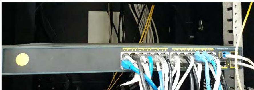
*Figura 21. Switch Cisco Catalyst 2960*
